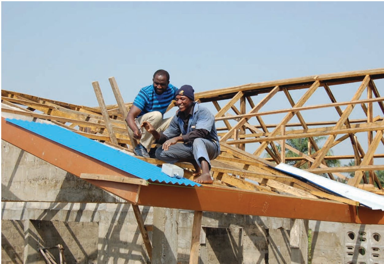
Adding zinc roof to the Three Communities Primary School
