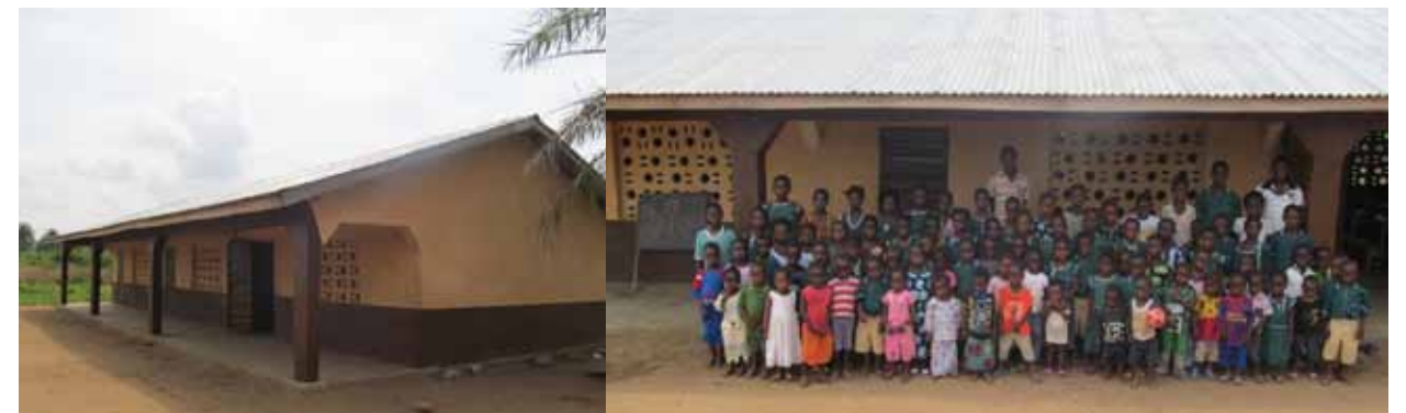
Tumba Primary School Completed in 2012
